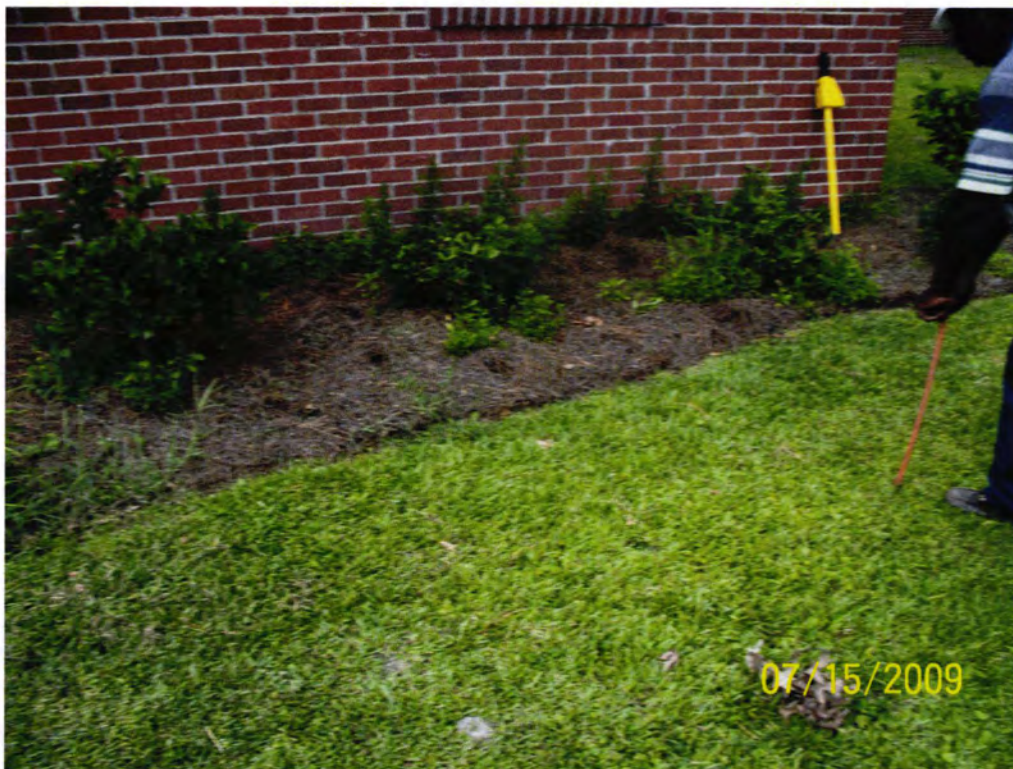
Picture 1: Location of UST 1392Dove prior to removal.
